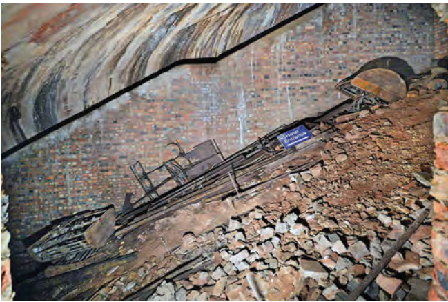
Section near the top of the railway that was not used in the war due to its proximity to the surface, looking through a post-war viewing opening through the stair side blast wall
